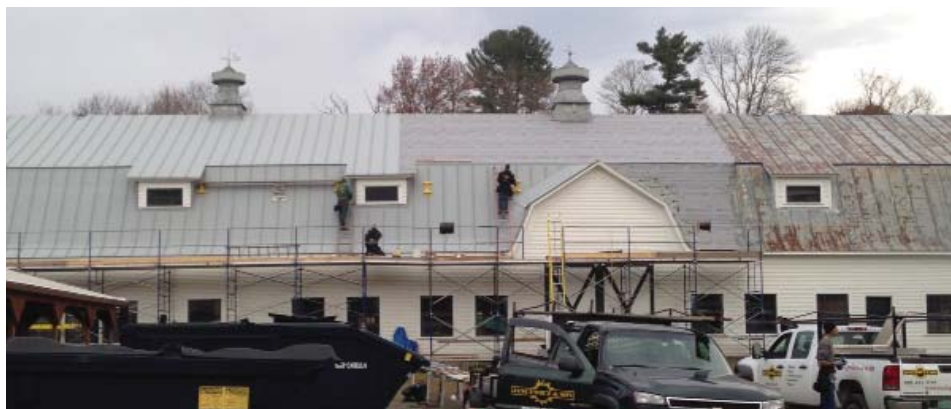
Our roof replacement project is now underway as of November 10, 2015.
